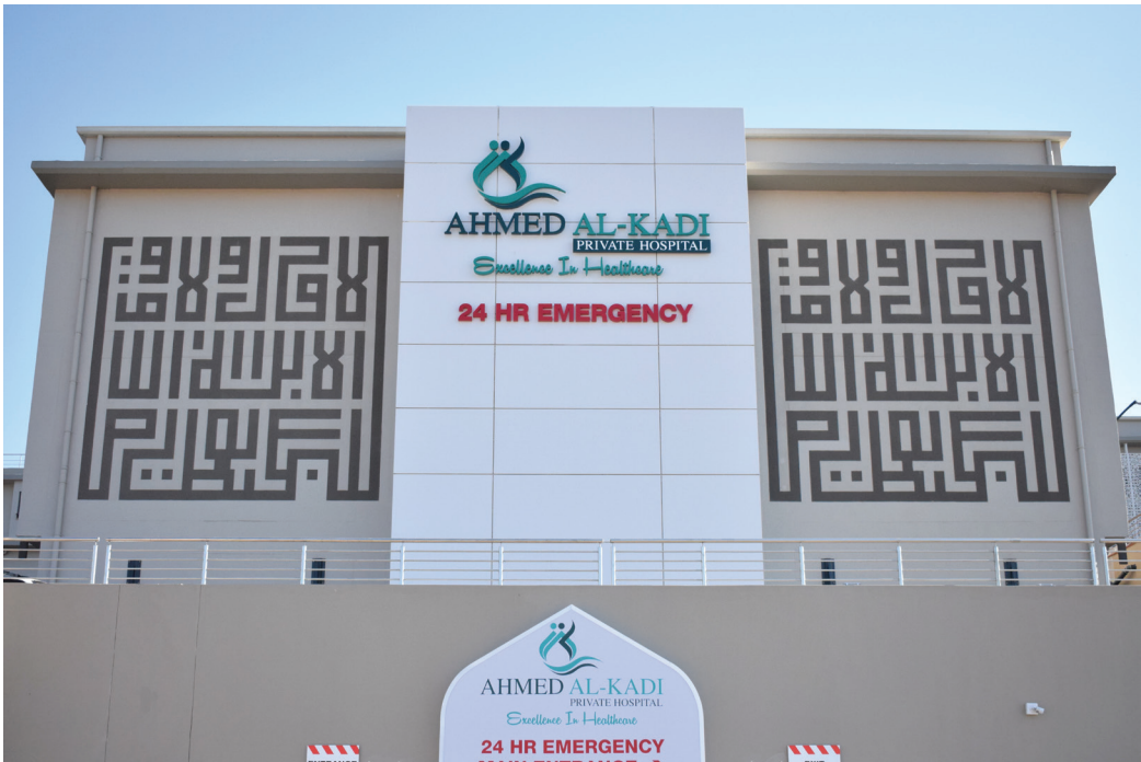
Ahmed Al-Kadi Private Hospital Waterfall Road main entrance
